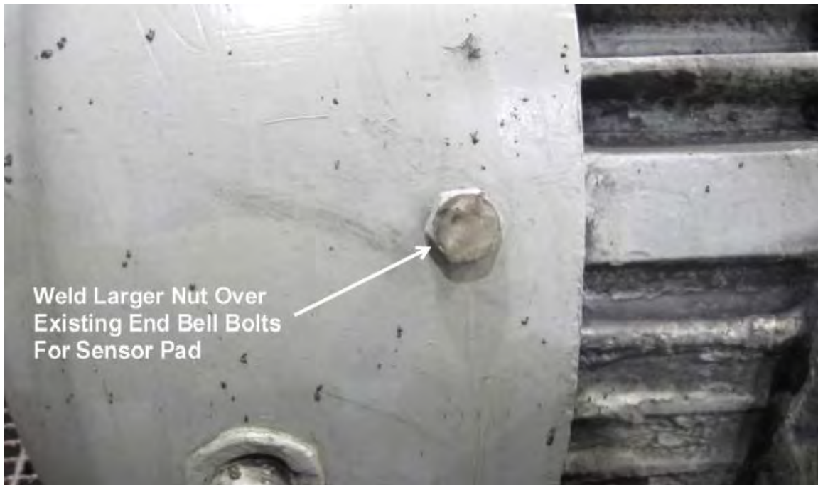
Figure 7 Larger nut head welded to existing smaller end bell
