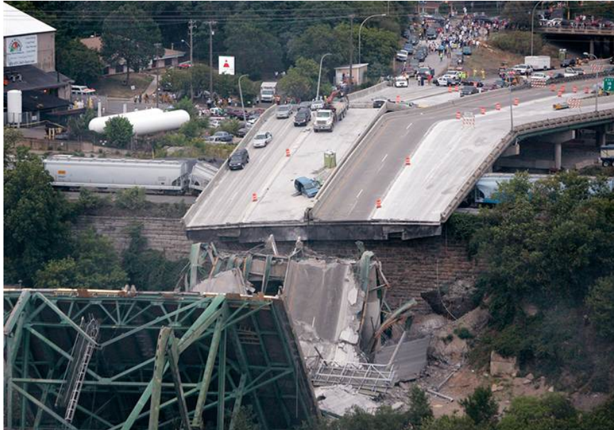
Figure 1: Photo of Minnesota bridge collapse [2]
