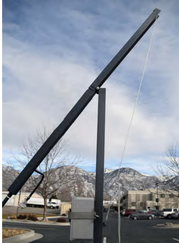
Figure 3-14 Pole in tip-down position
