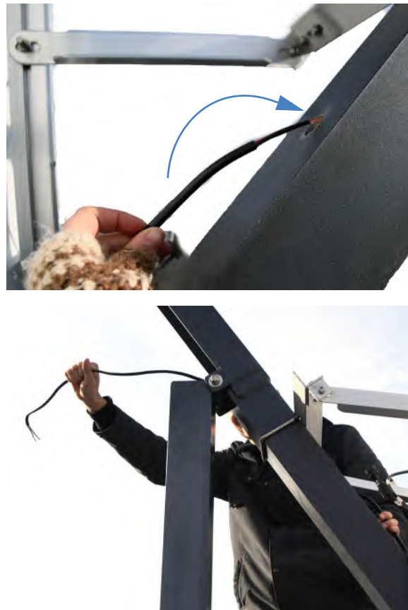
FIGURE 4-2 Feed Cable Down Pole
