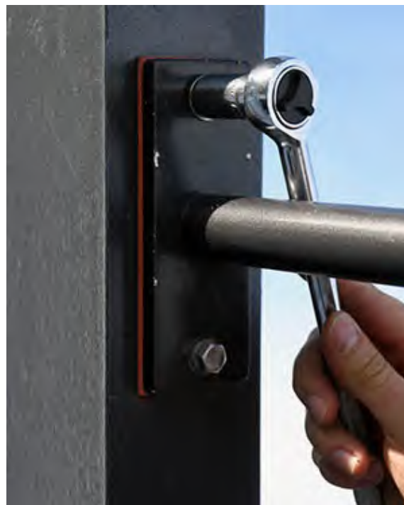
FIGURE 4-16 Weather Arm Bolted to the Pole
