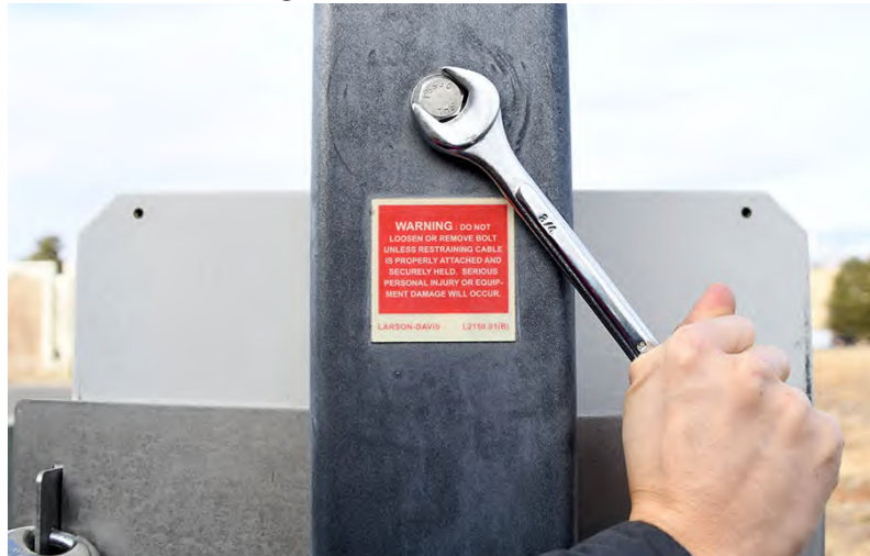
Figure 3-13 Removing Bolt from Pole
