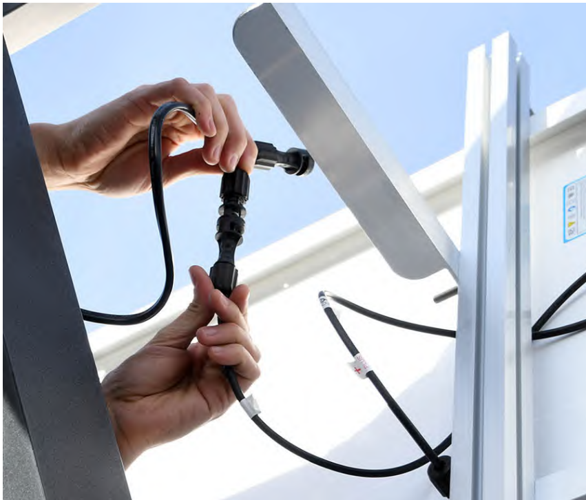
FIGURE 4-4 Connect Solar Cable to Panel
