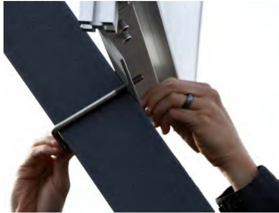
FIGURE 4-1 Solar Panel Install
