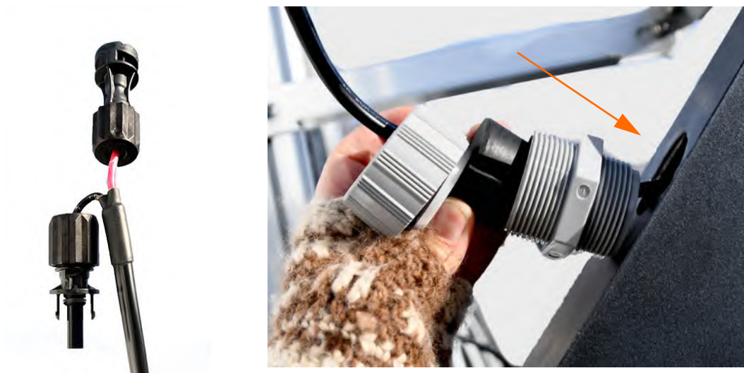
FIGURE 4-3 Gland Install
