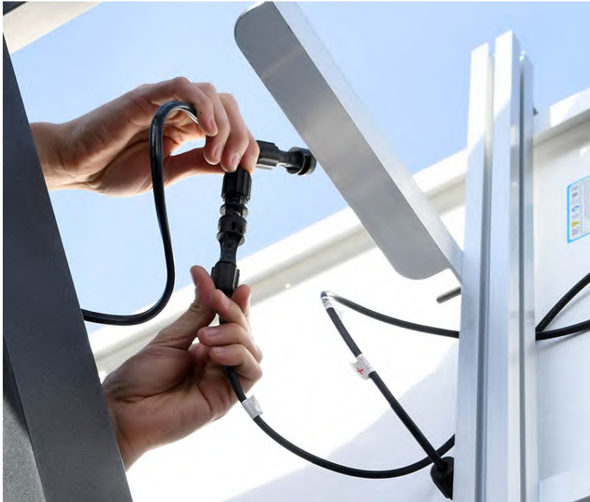
FIGURE 4-11 Connect Solar Cable to Panel
